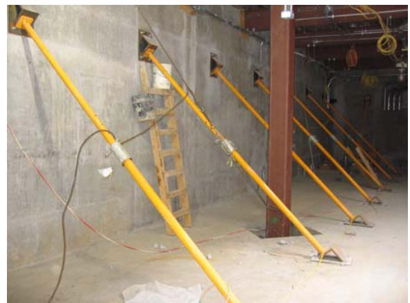
Figure 7. Shear Wall Support
