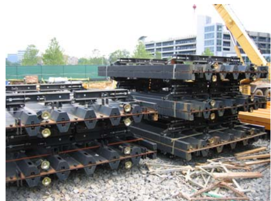
Figure 4. Ulma Forms in Staging Area
