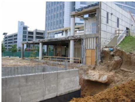
Figure 3. Base Building Demolition
